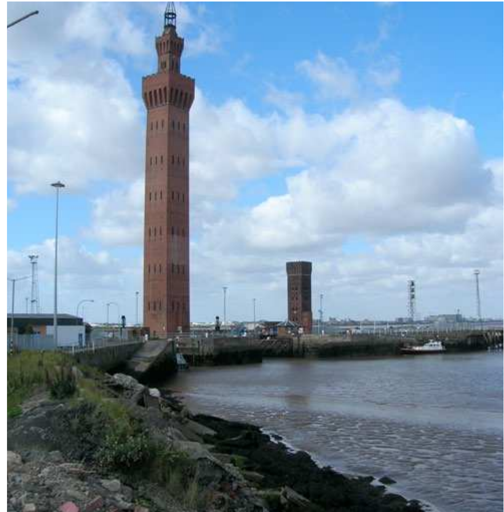
Grimsby Dock Tower is a prominent feature on the docks with modern infrastructure now dominating the skyline.
